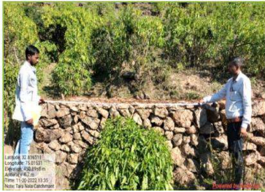
Photo-7: Measurement of SMC work- Crate
