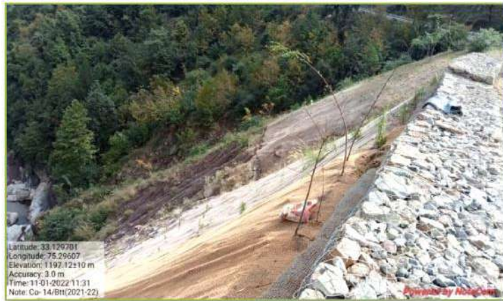
Photo-19: Jute mat at Batote NH1A plantation site
